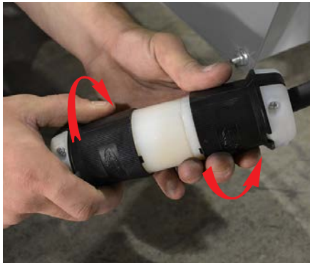
Twist connectors to lock in place
